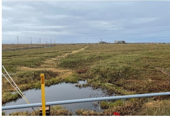
Figure 10: Trenching damage looking south toward the old Air Force hangar. Tracie Curry 2022.
