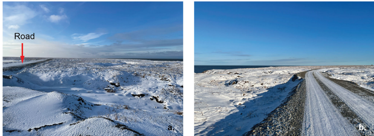
Figure 2: Erosion undercutting North Road (70° 7'57.05"N, 143°40'11.27"W). (a) Facing West. (b) Facing East.
