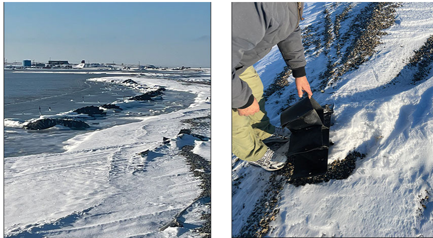
Figure 3: (a). Degraded shoreline protection on the southern edge of the spit. (b). Close-up of degraded plastic material
